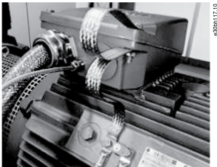
Illustration 10: Installation of EMC straps from the Terminal Box to the Motor Frame
