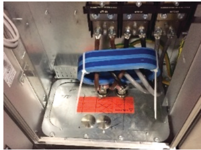
Fig. 6.21 Common-mode cores installed at the drive terminals
